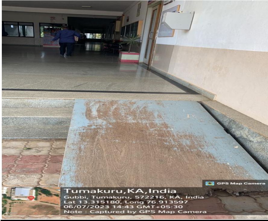
Ramp Near CRC Block
